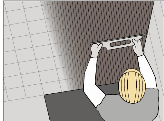
Spread adhesive on the existing substrate
